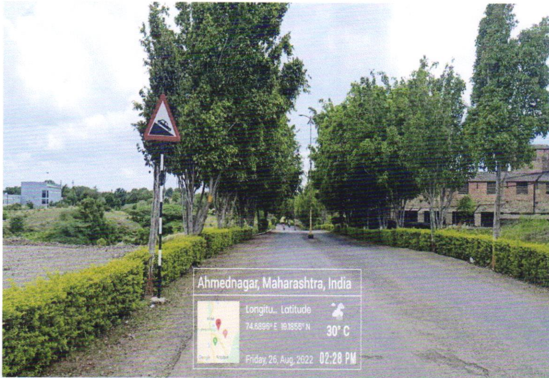
Steep Descent sinage
